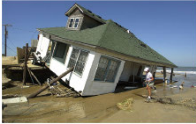
flood loads compromise foundation
