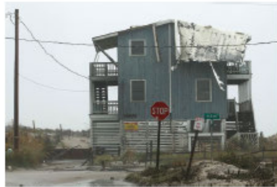
low-slope roof subject to uplift damage
