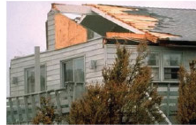
improper nailing (often due to nail gun usage)
